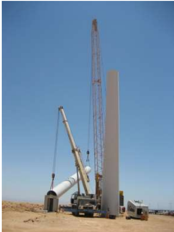
Figure 1.8: Activities due to wind turbine erection
