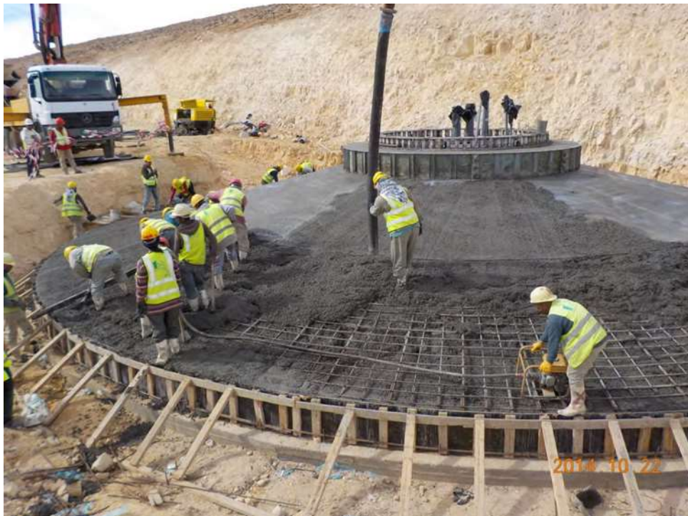
Figure 1.7: Example of a wind turbine foundation
