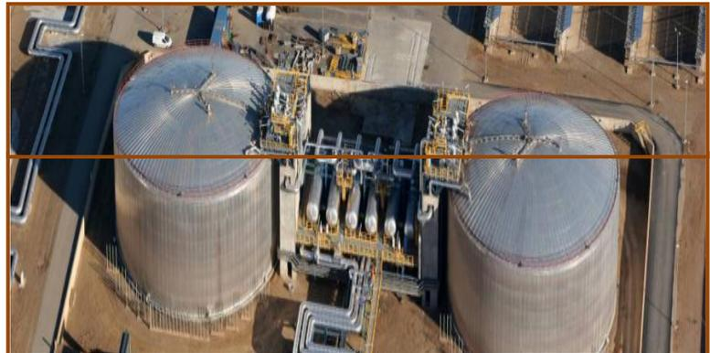
from the hot tank to generate enough steam to generate electricity at night from 4-6 hrs to share in cover the peak load at night .
