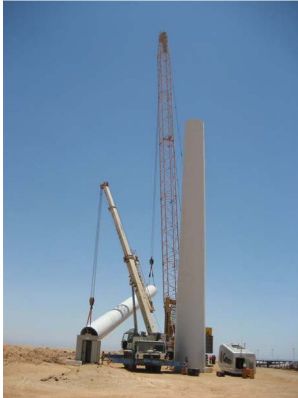
Figure 1.8: Activities due to wind turbine erection
