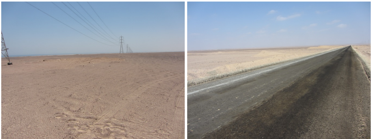
Figure 4.75: 220 KV overhead powerline at the eastern border of the project area (left) and track for wind farm development (right)
