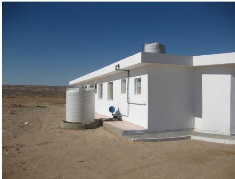
Figure 1.11: Typical temporary office facility at a wind farm site used during the construction phase
