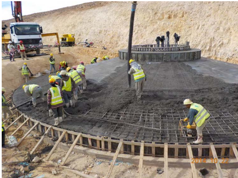
Figure 1.7: Example of a wind turbine foundation
